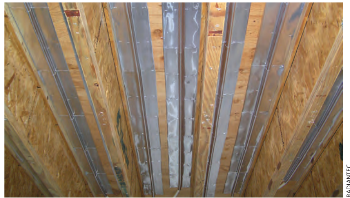
Aluminum heat-emission plates, like the homemade plates shown above, are sized to fit between floor joists. One or two grooves bent into the flat plate accommodate pex tubing.
