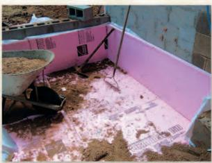
A gridwork of PEX tubing is installed in the lower portions of the sand bed. Solar-heated fluid pumped through the gridwork of tubing heats the sand. Heat then radiates from the sand through the floor and into the building.
